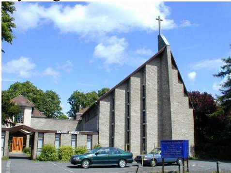
Arbury Road Baptist Church, Cambridge
